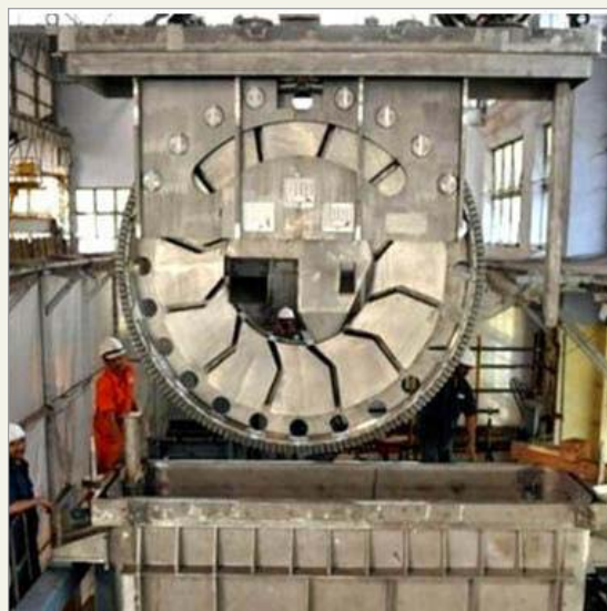
Fig. 2 Plant scale CRD during installation
